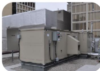
An encased unit to be fitted into the HVAC/AHU unit or the air ducting to provide an airtight flow of the airstream through the unit and has the option for a removable **MERV-13** and **Activated Charcoal (ACF) Filter**. This model consists of three photocatalytic grids to provide additional dwelling time for maximum breakup of the molecular structure of the VOCs passing in the airstream.
