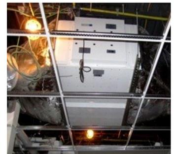
Using a high proportion of return air as part of the airstream (between 85% to 95%) is thus helping in this cleaning process, as the recirculating return air already passed before through this photo-catalytic oxidation process. Recirculation of the airstream is also a very important concept for saving energy as already conditioned for the required room temperature.
